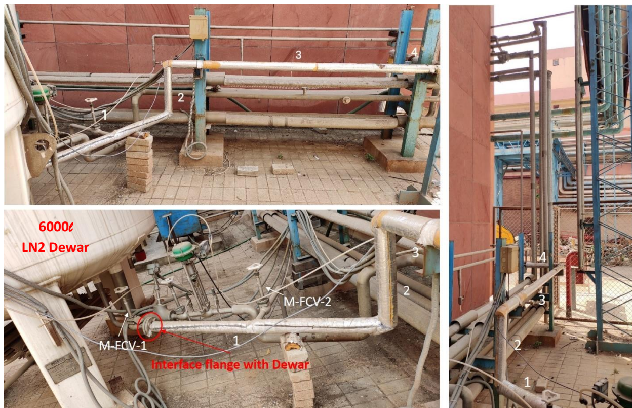
Figure 9: Physical Interface with 6000 l LN2 Dewar
