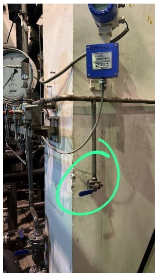
Figure 5: Compressed Air Line Source Point
